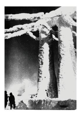
Figure 1- Condition of a transmission line after a snow storm in Paylodar oblast
