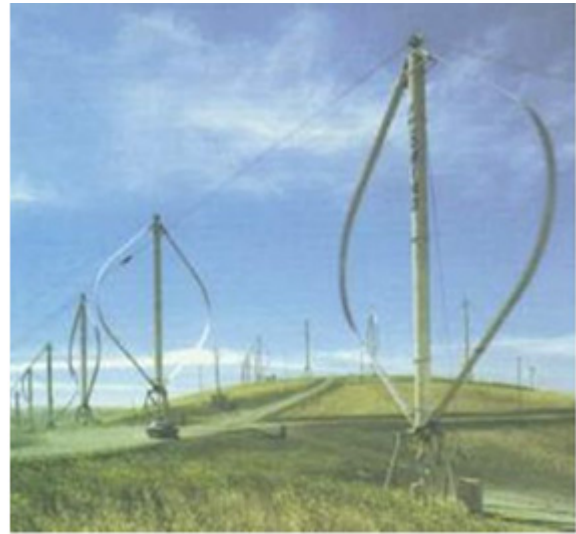
Figure 1 – Wind turbine with the turbine to Darrieus of system troposcino
